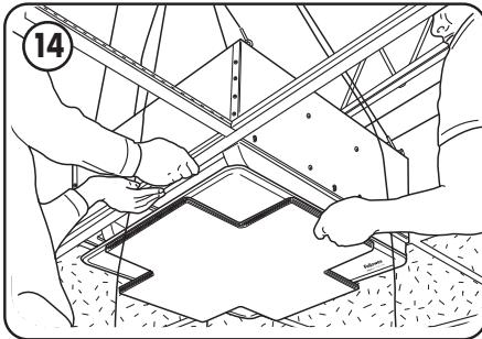
With one person supporting fixture so it just touches the grid, the other should pull the aircraft cables until taut.
